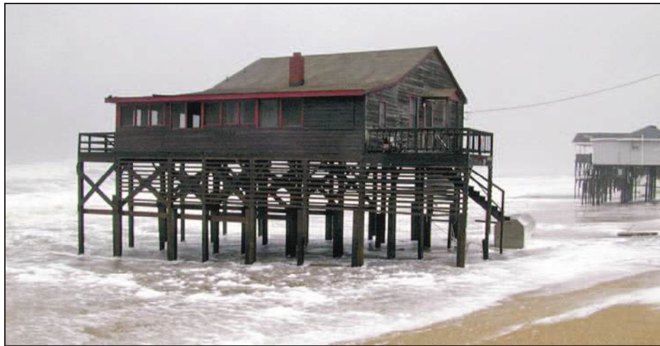
Figure 4-3. Long-term erosion left this well-built Kitty Hawk, NC, house standing in the ocean (Hurricane Dennis, 1999)
